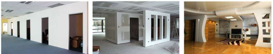
Partitions and Drylining
